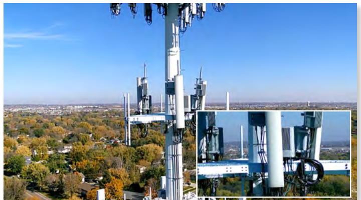
Livestreamed 4K Video Actual screen capture of tower inspection
